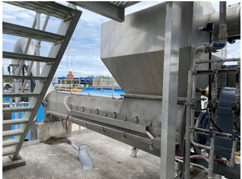
Figure 4 – A Screw Wash Press at a treatment plant is very similar in shape and mechanism to the crusher-destemmer
