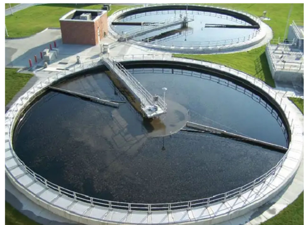
Figure 10 – A typical clarifier arrangement
