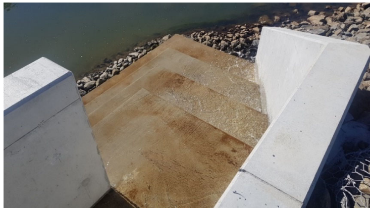
Figure 16: An outfall of a treatment plant showing the final treated effluent – Almost good enough to drink.
